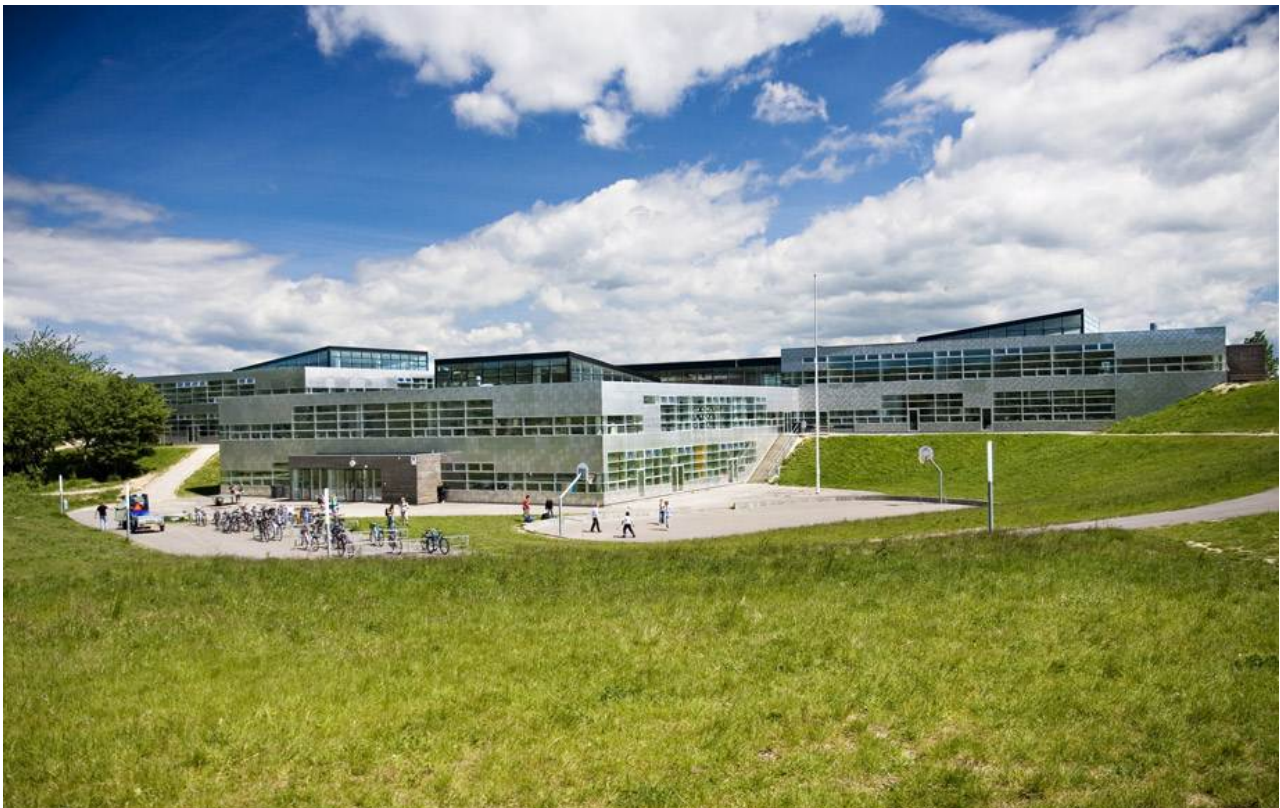
Figure 3: Absalon School. External view
