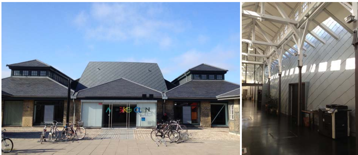
Figure 1: Music School with the concert hall, exterior and internal view of covering
