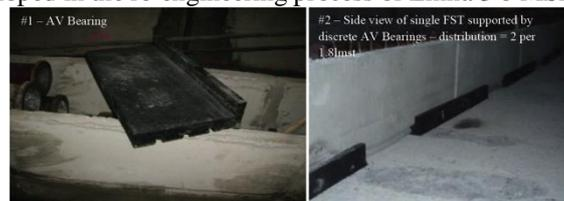
Figure 5 : Details of FST with discrete AV bearings
