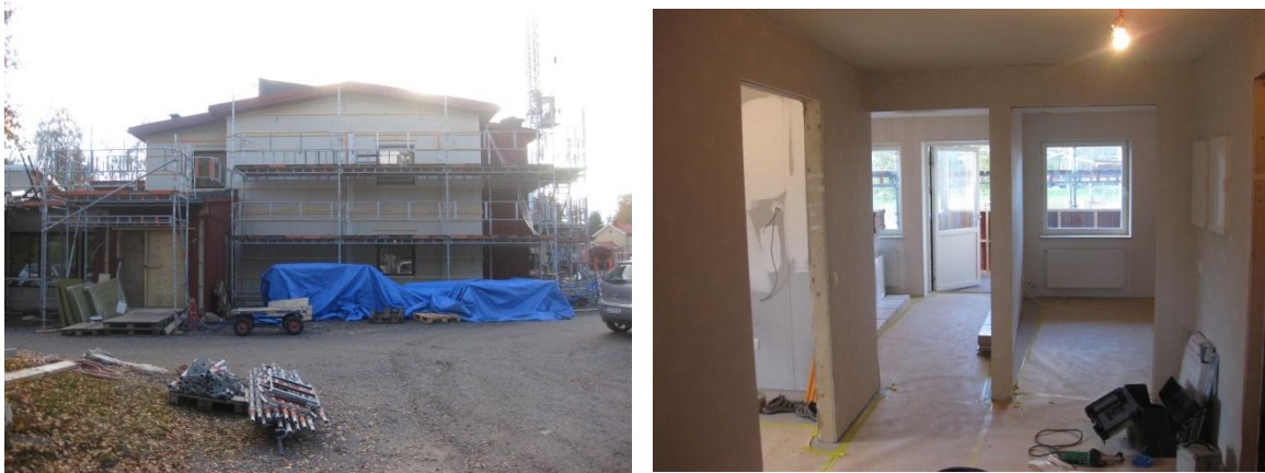
Figure 1: The building and measured dwelling.
